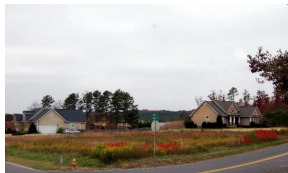
Single family residential housing on Cohutta-Varnell Road
