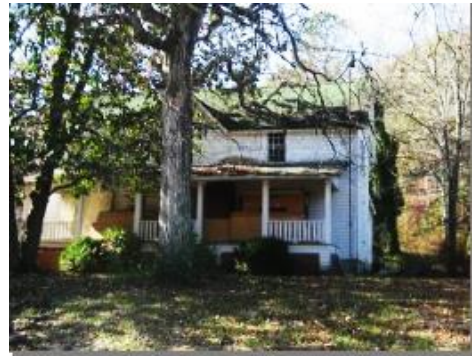
Another example of the Rural Neighborhood Revitalization character area in southeast Whitfield County
