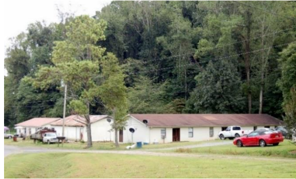
Multi-family residential housing on Mount Olivet Drive
