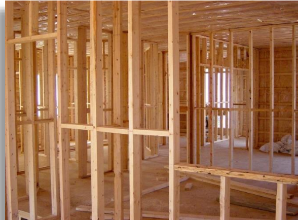
Figure 31: A community with a thriving housing market creates employment opportunities for skilled laborers and entrepreneurs needed to create the supply of housing stock
