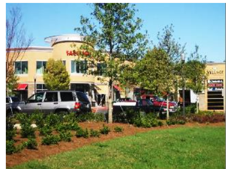
Quality commercial development shown here from the Town Center area of Cobb County, Georgia
