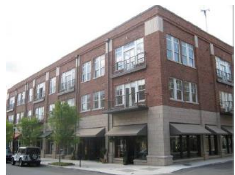
All new construction should contribute to the existing historic commercial character
