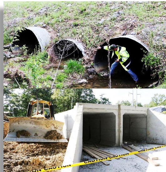
Figure 36: Before and after of a culvert replacement on Beaverdale Rd. where Whitfield County saved approximately $300,00 by utilizing its on public works department rather than a contractor
